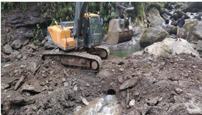
Figure 7- 2: Cross drainagae constuction at Kitchhe Khola
