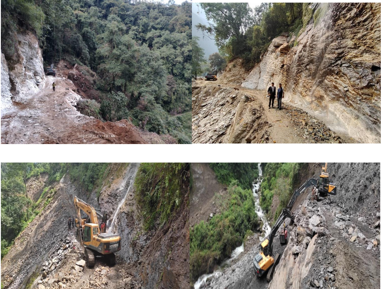
Figure 7- 1: Road construction and surface grading ongoing and mucking after blast at Chainage 3+800
