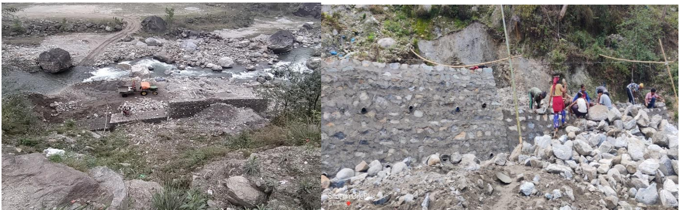
Figure 5- 1: Protection work construction is in progress
